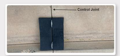
ALIGN THE RAMP SET WITH THE JOINT
